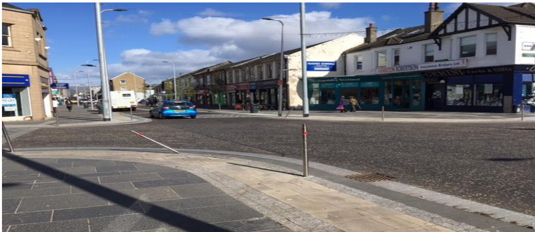
Photographs 13 Illustrating the tactile used at informal crossings with none extending to building line at informal crossing on Cowgate Street.
