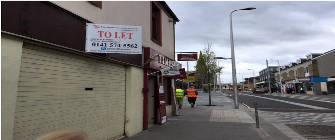
Photographs 13 Illustrating the tactile used at informal crossings with none extending to building line at informal crossing on Cowgate Street.
