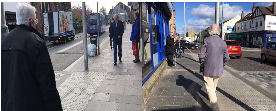
Photographs 11 and 12 Illustrating the tactile used at informal crossings with none extending to building line on Cowgate, at the Catherine Street / Kerr Street junction
