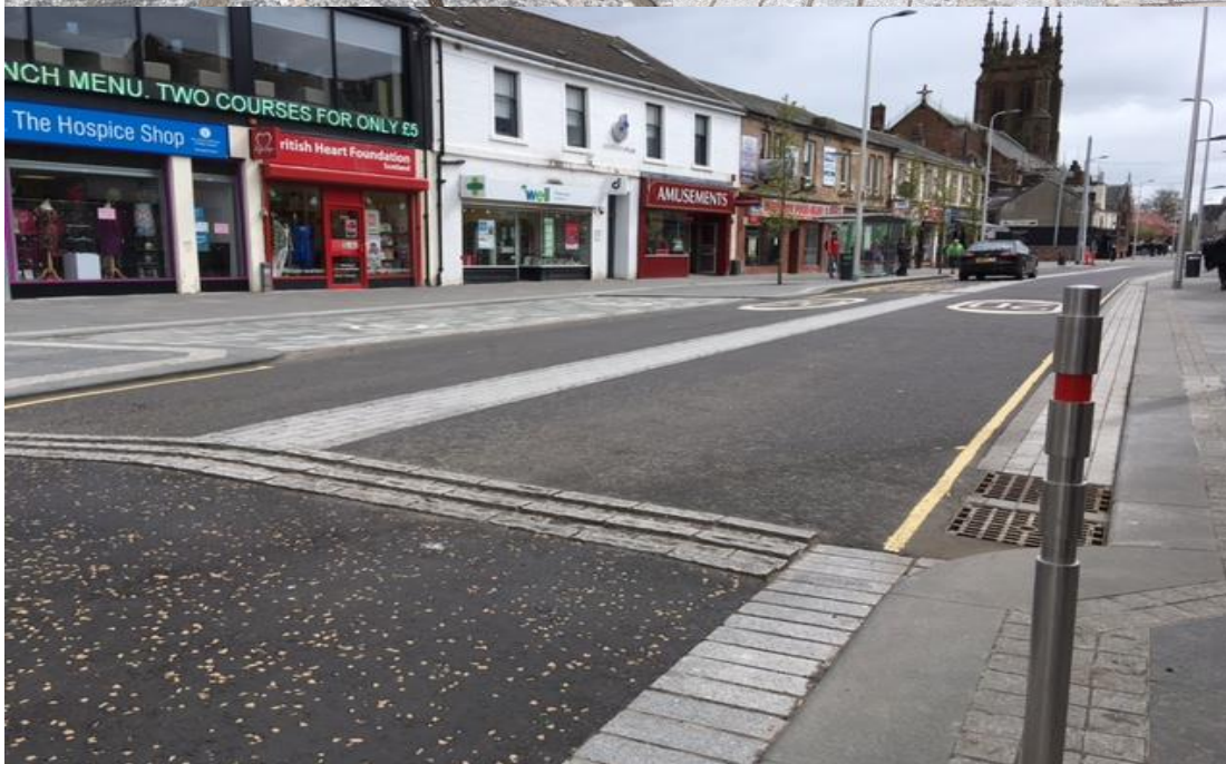
Photographs 17 to 19 illustrate the upturned bricks along Cowgate Street
